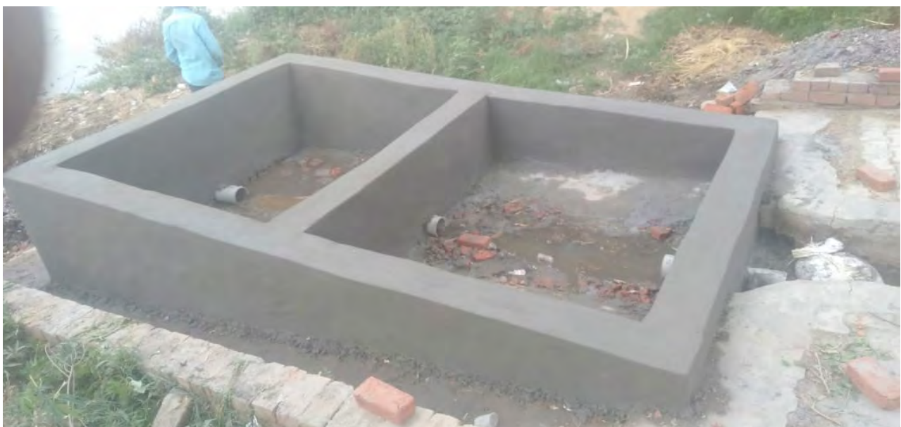
Structure of Filter tank in BadaTalab, KacheraVarsabad
