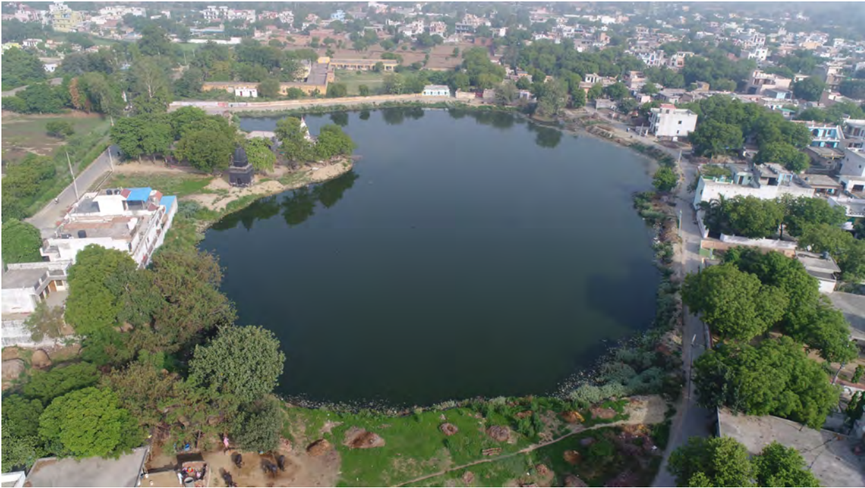
Tank near Govt Primary School in Dujana after DA's Intervention
